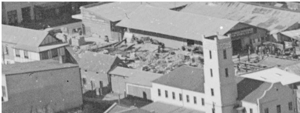
Figure 2.59 Detail from EW Searle's oblique aerial of Parramatta, c1939/1940, showing Lots 2 and 3 of Allotment 16 as vacant land. The building material on the site could be debris left over from the fire which destroyed the old Victoria Theatre in May 1939. It could also be site material for the construction of the shops in 1930. (Source: National Library of Australia)
