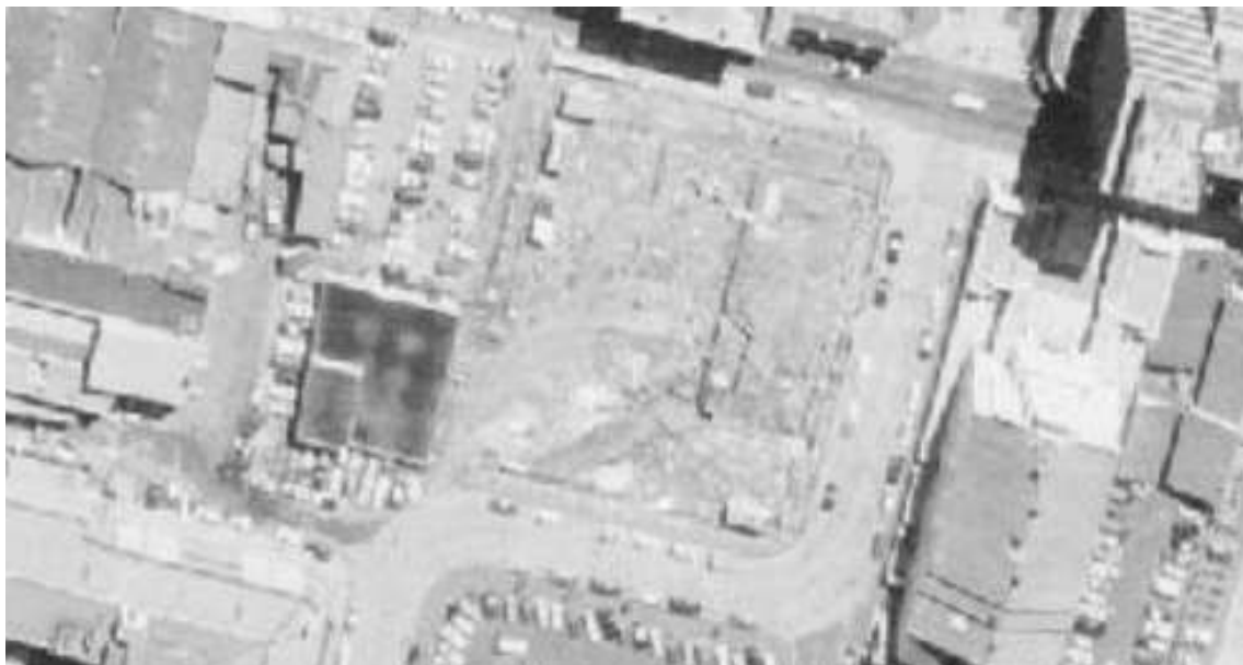
Figure 4.50 1978 aerial photograph during construction of Parramall. (Source: NSW Spatial Portal img 2707–13–144)
