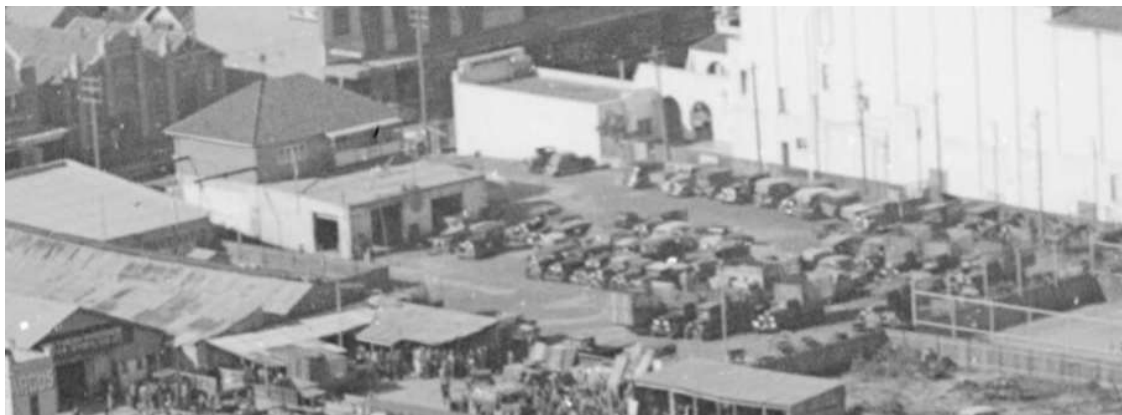
Figure 2.25 View from southwest to Roxy Parking and Service Station, about 1935. (Source: NLA)
