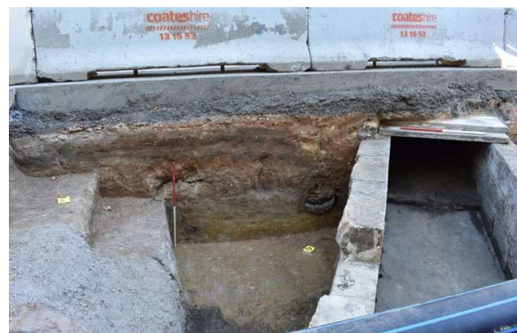
Figure 4.36 Northeast-facing section showing levelling fills on the eastern side of the drain. Excavation in the northern (eastbound) lane of Macquarie Street. (Source: GML 2020)
