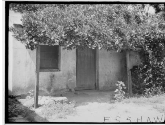
Figure 2.165 Rear view of Margaret Houison's house, Macquarie Street, 1931, photographed by EG Shaw. (Source: State Library of NSW)
