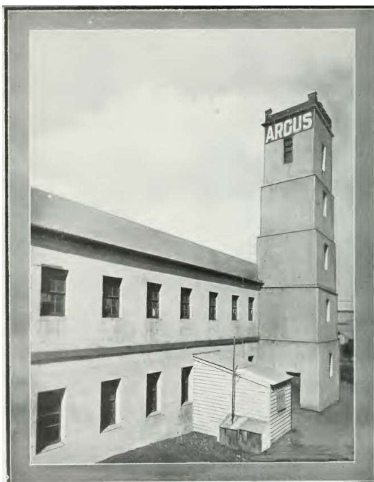
Figure 2.123 The Cumberland Argus Printing Works, Parramatta, on land at the rear of Macquarie Street (Allotment 81). (Source: Wharton, JC 1911, The Jubilee History of Parramatta , Cumberland Argus, Parramatta, p 146)
