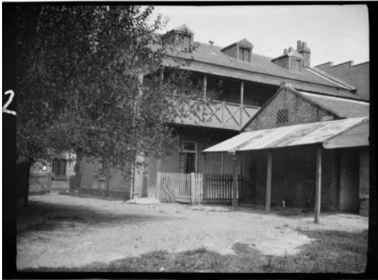
Figure 2.164 Rear view of Margaret Houison's house, Macquarie Street, 1931, photographed by EG Shaw. (Source: State Library of NSW)
