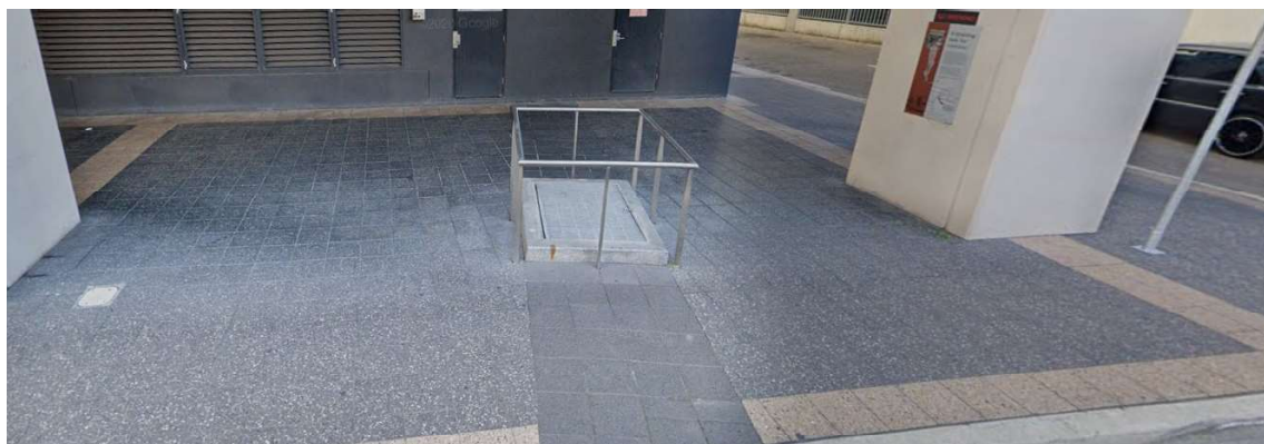
Figure 4.37 The location of the conserved section of Town Drain at the northwest corner of 25 Smith Street and 76–78 Macquarie Street, marked by different coloured paving tiles. (Source: Google Maps Street View, accessed 15 July 2021)
