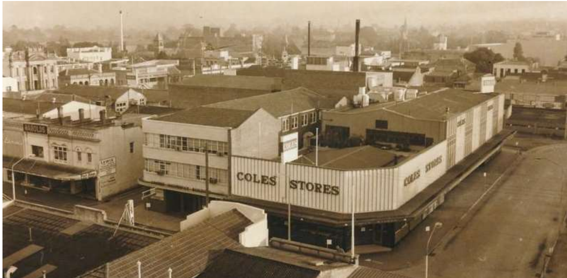
Figure 2.138 Coles Store and United Insurance Building, Macquarie Street, 1968. (Source: City of Parramatta Research & Collections, ACC209/016)
