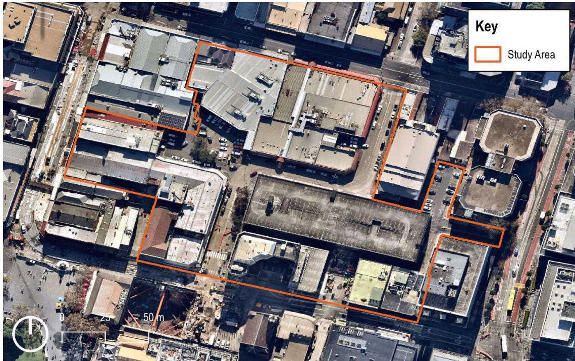
Figure ES1 The Parramatta metro station construction site in its immediate context. (Source: GML 2021, with Sydney Metro data, over base map from Nearmap)
