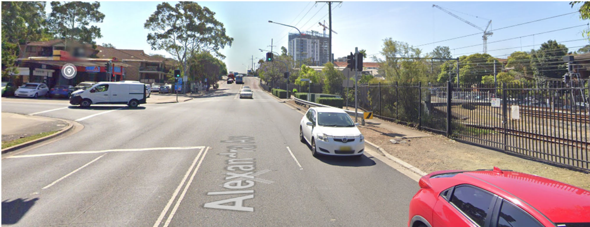
Figure 2-9: Rail corridor access gate
