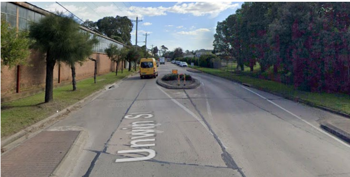
Figure 5-7: Speed management device on Unwin Street
