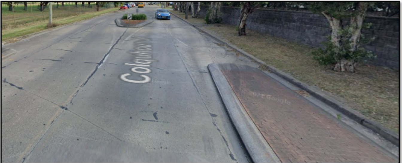
Figure 5-8: Speed management device on Colquhoun Street
