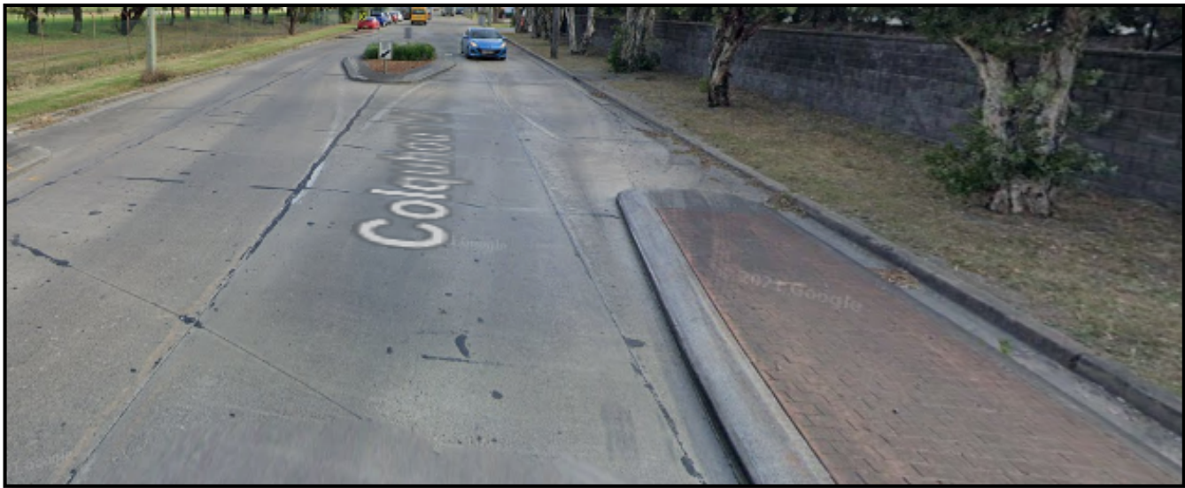
Figure 5-8: Speed management device on Colquhoun Street
