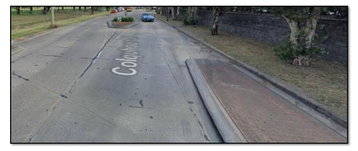
Figure 2-9: Speed management device on Colquhoun Street
