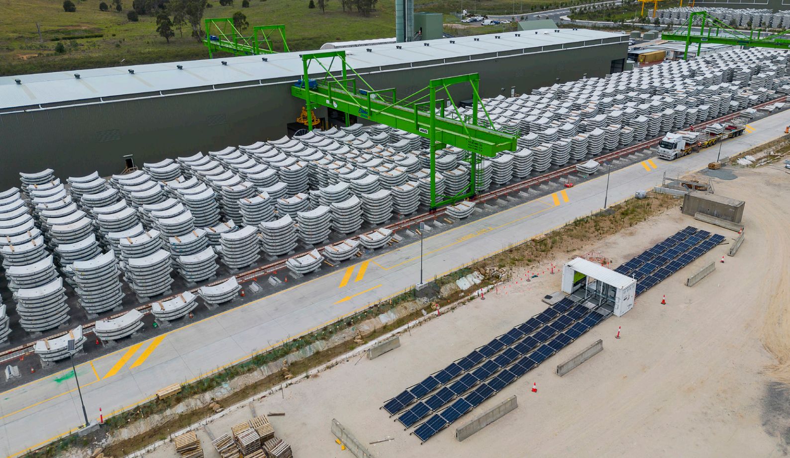
A 20kWp mobile solar farm supplements the Eastern Creek Precast facility's electricity needs.
