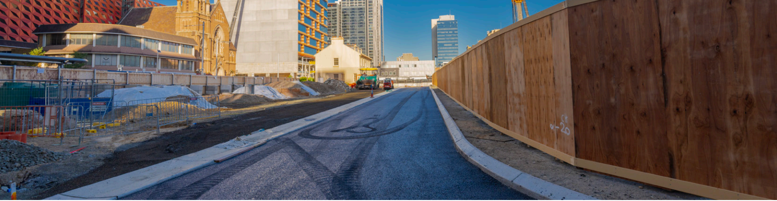
Reconophalt lay in progress at the Project's Parramatta metro station site.
