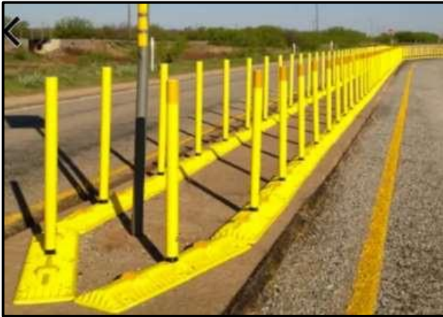
Figure 3-19: Temporary kerb delineation
