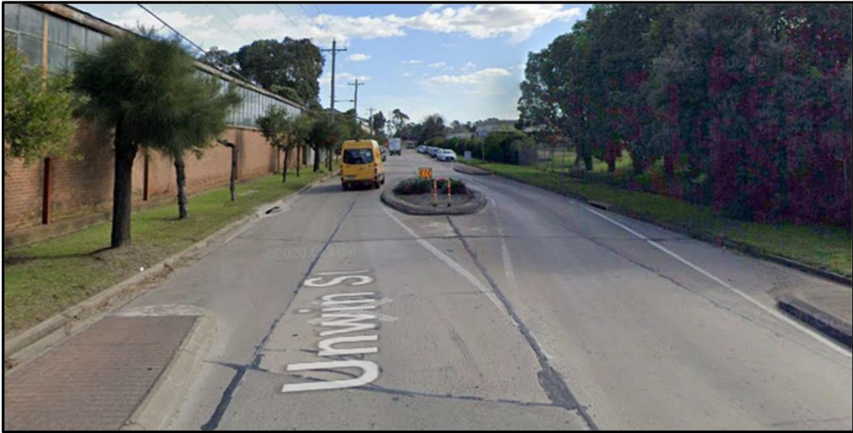
Figure 2-7: Speed management device on Unwin Street
