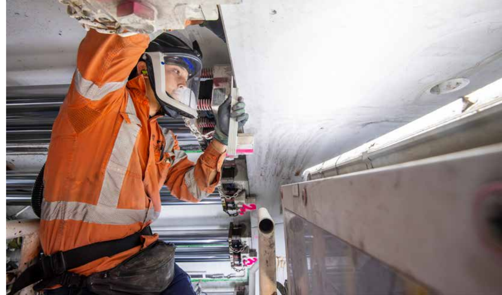
Installation of segment rings on TBM Dorothy
