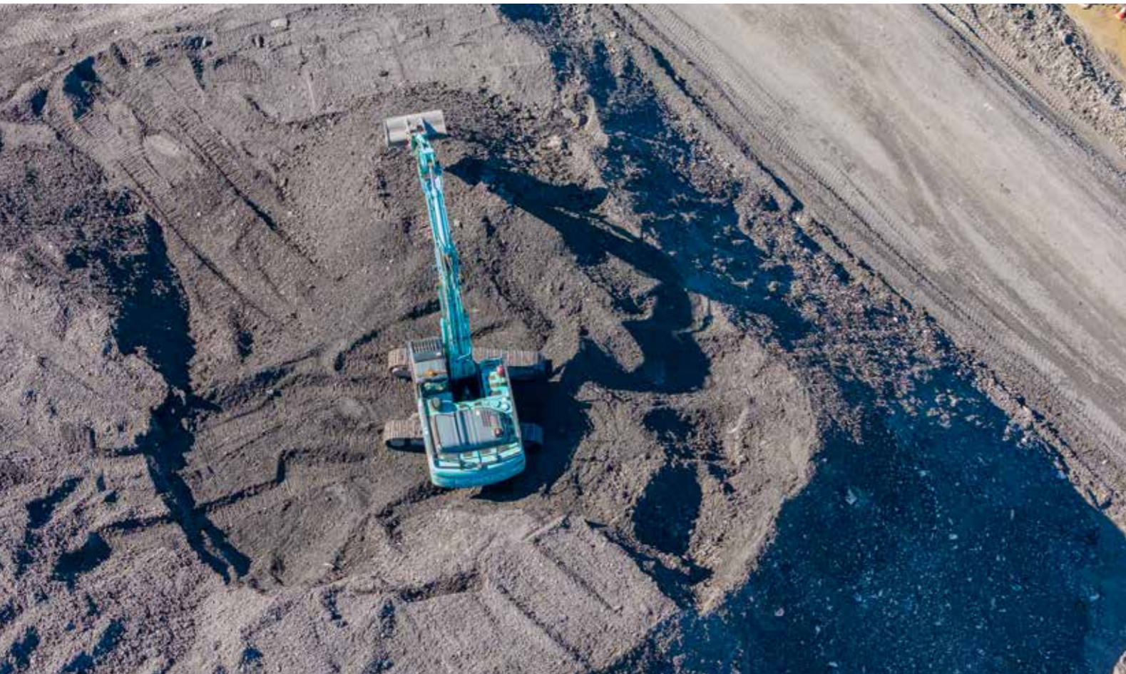
Earthworks at the future stabling and maintenance Facility in Clyde
