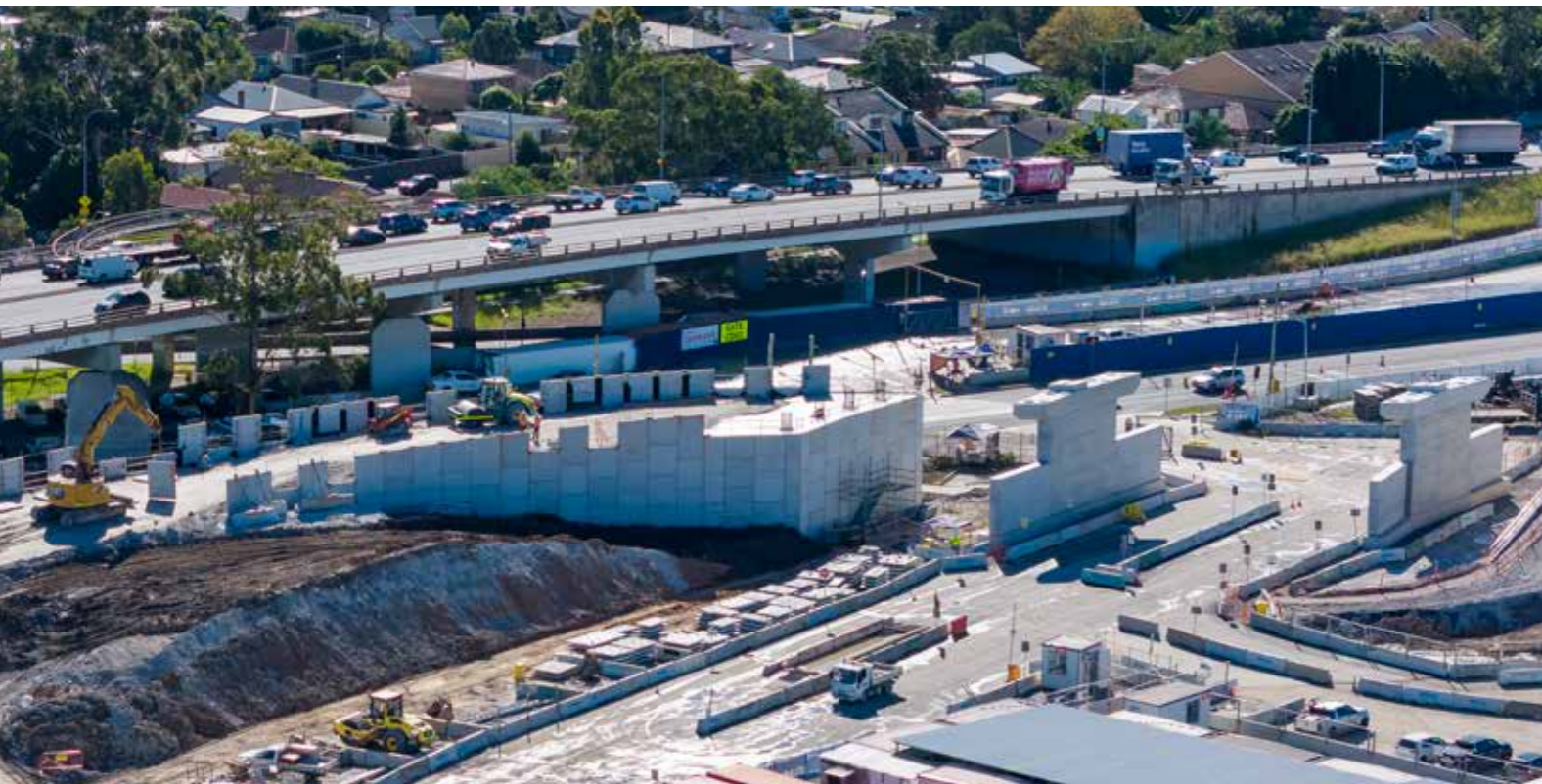
Unwin Street civil work
