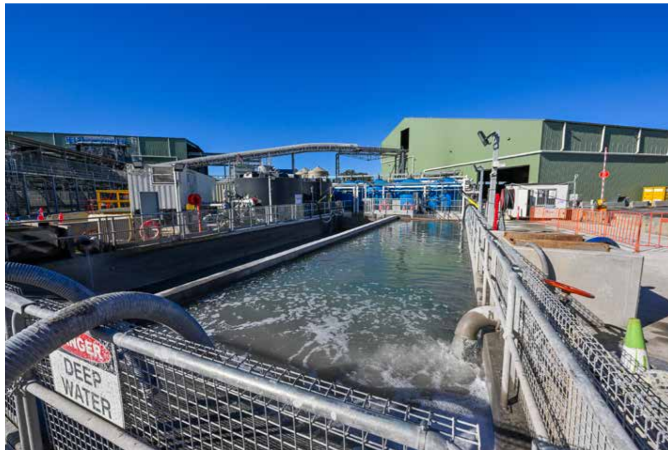
Water Treatment Plant at the Rosehill site
