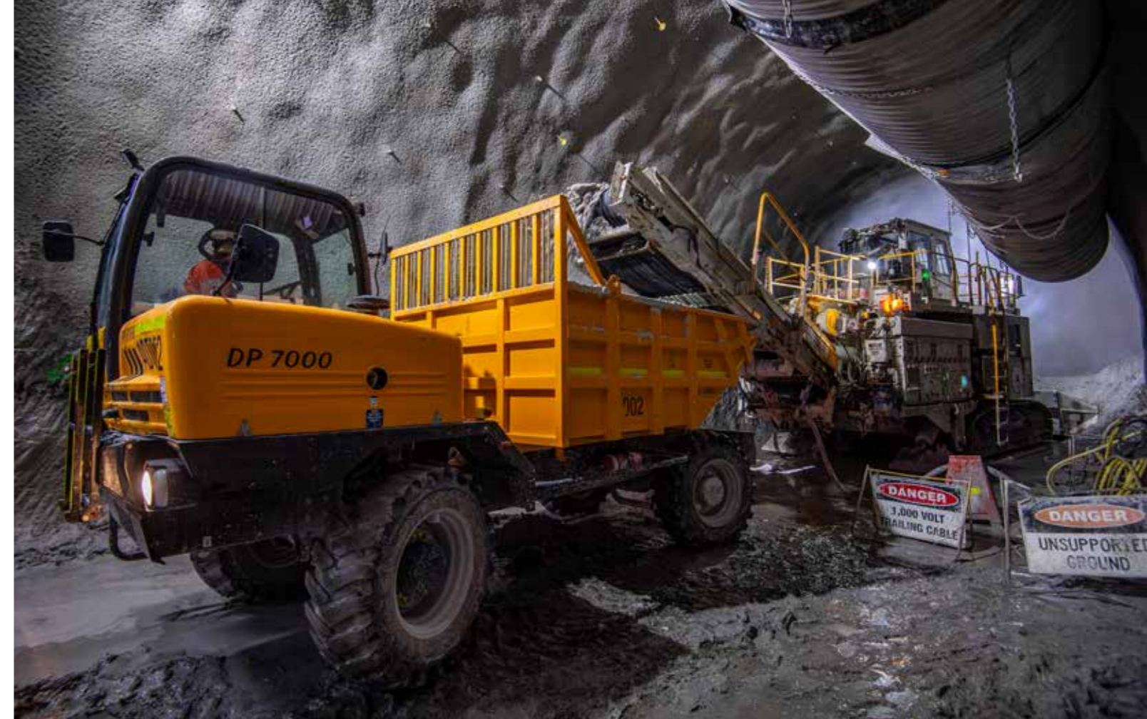
Roadheader in the Clyde Dive service tunnels
