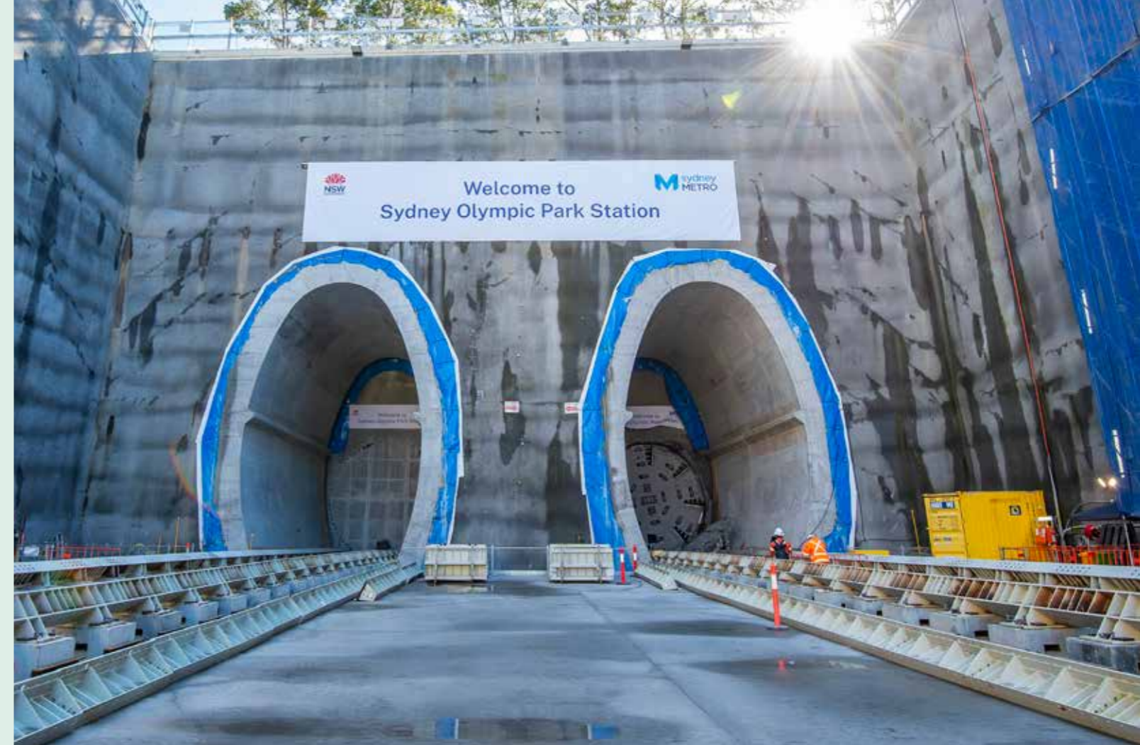
TBM Betty arrives at Sydney Olympic Park in June 2024
